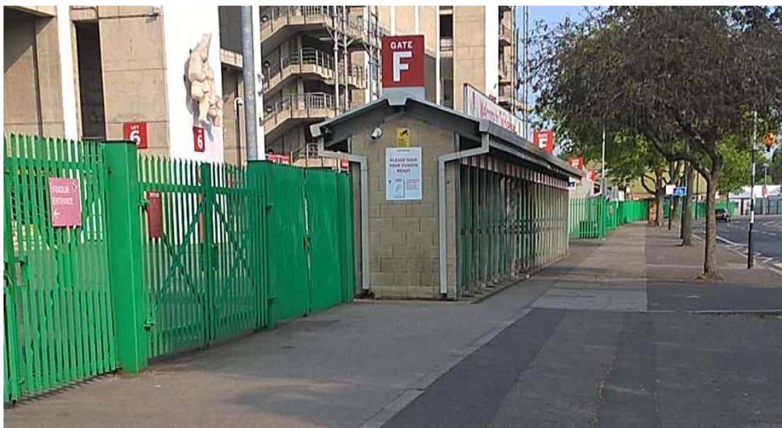
Fig. 3 Turnstiles to be maintained
