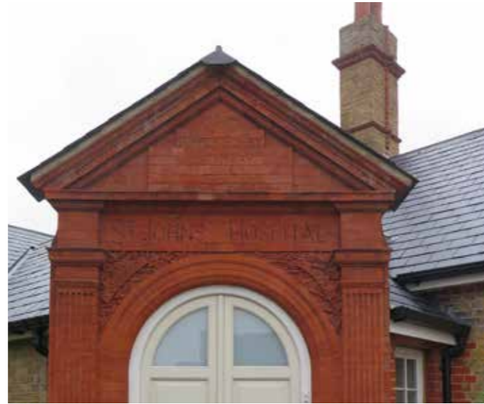
Fine moulded brickwork at former St. John's Hospital, 58 Amyand Park Road
