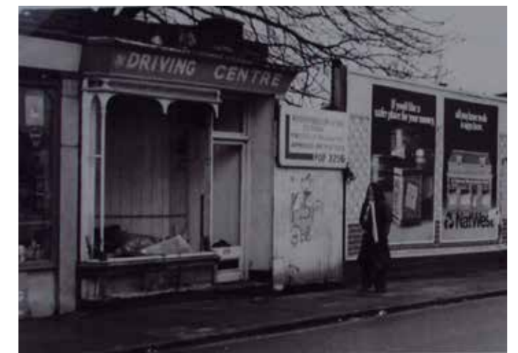
Station Approach, looking towards railway line and station yard, 1978
