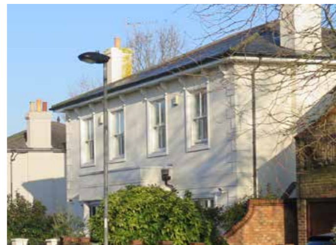
Two-storey villas to the east of Belmont Road
