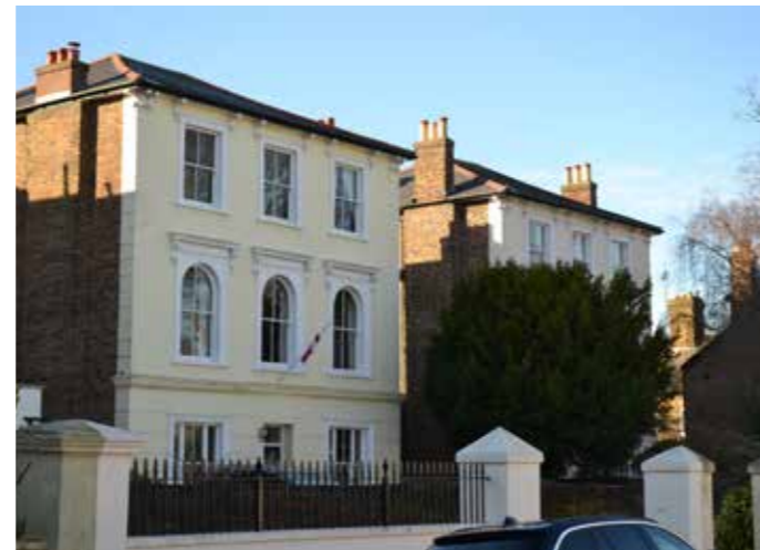
Large three-storey villas on the west side
