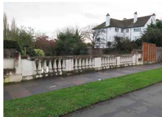
Chertsey Road bridge
