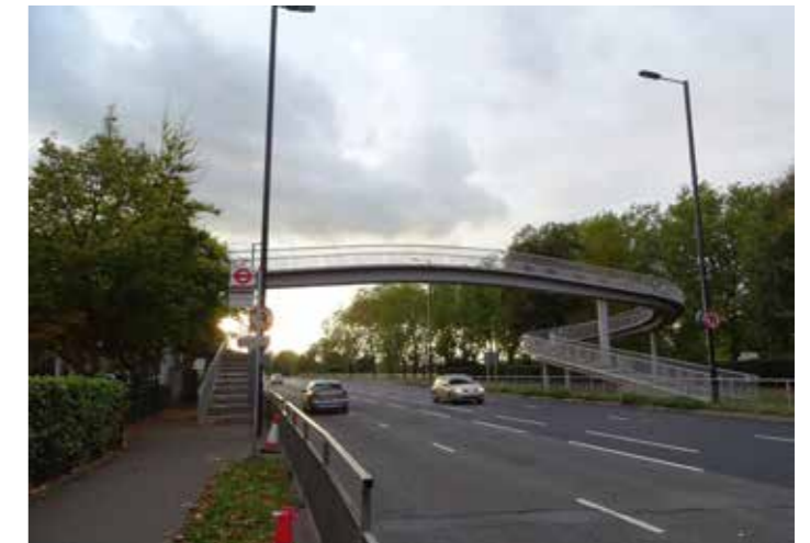
Footbridge over A316
