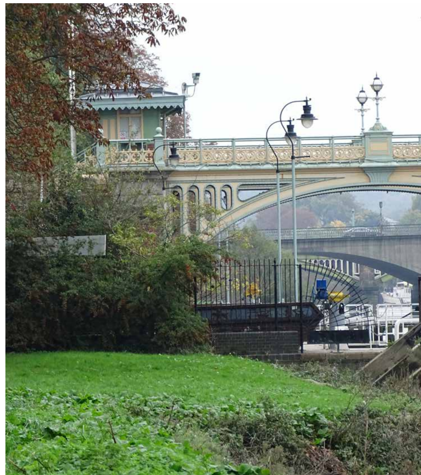
Richmond Lock footbridge, Twickenham Bridge and Richmond Railway Bridge
