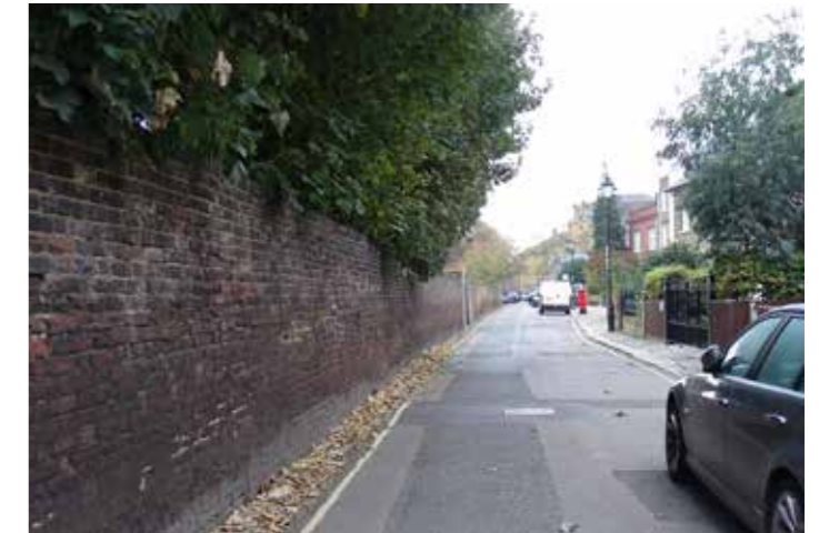
Kew Foot Road boundary wall
