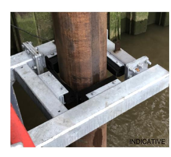
**EZ DOCK PILES AND PILE GUIDE** UNTREATED STEEL PILES AND PILES GUIDES (PONTOONS NOT AS SHOWN)
