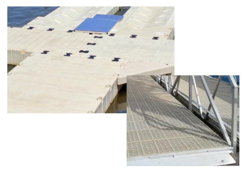
**EZ DOCK PONTOON WALKWAY AND GANGWAY** BUFF COLOURED POLYSTER RESIN MODULAR PONOONS CONNECTED WITH ALUMINUM GANGWAYS COVERED WITH BUFF COLOURED GRP DECKING
