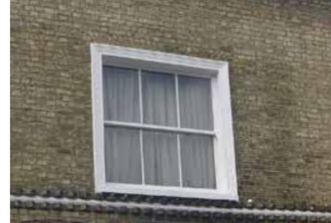
A Victorian three-light sash
