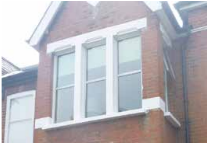
Replacement narrow bar uPVC windows filling three long openings in a late-Victorian bay
