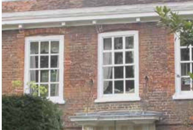
Georgian 'six over six' flush sash window
