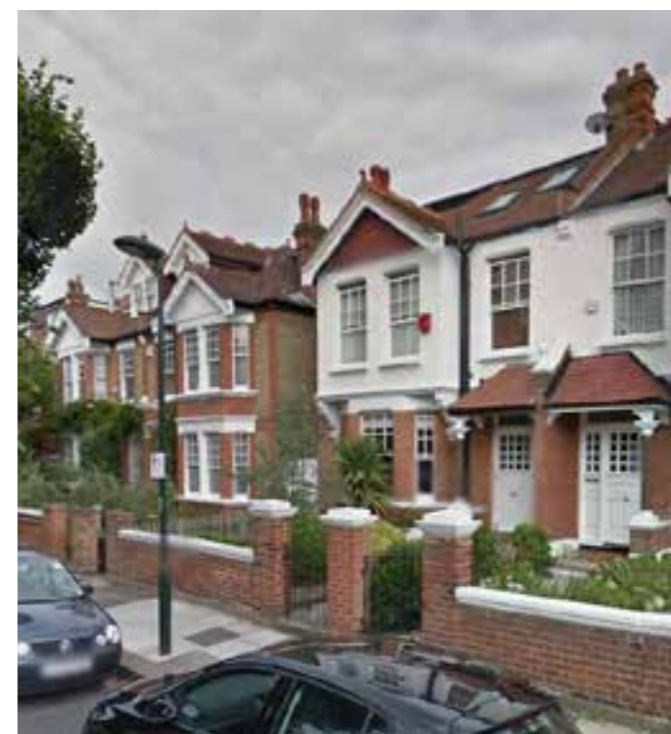
White capped walls and pillars - Westmoreland Road
