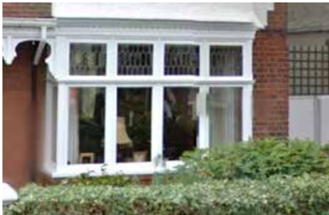
An Edwardian timber-frame hybrid bay window with leaded transoms
