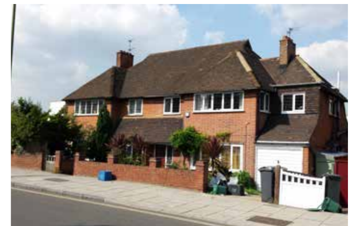
Upper Richmond Road West
