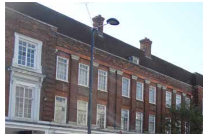
Interwar neo-Classical metal-framed windows
