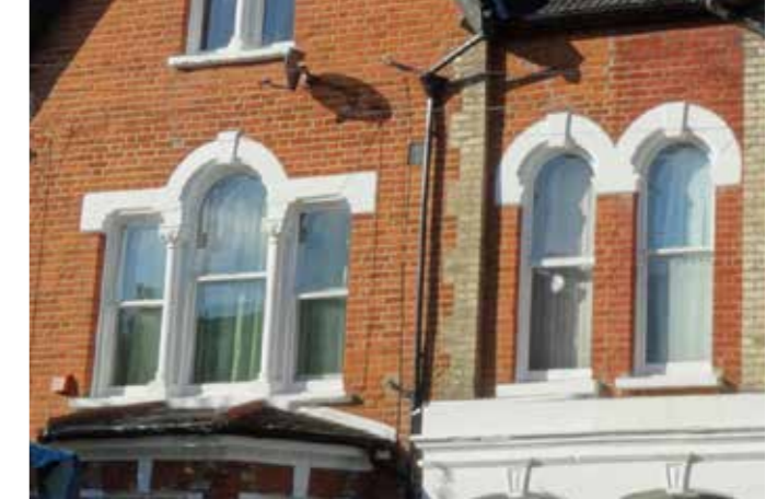
Victorian Classical sash windows with arched upper sash and decorative plasterwork column jambs
