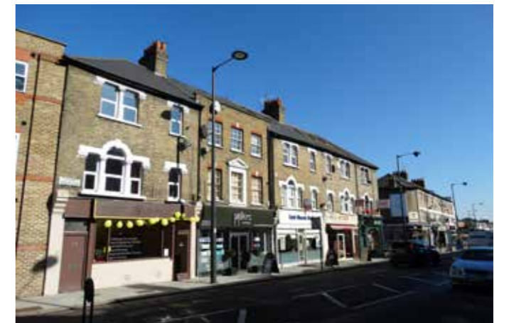
Upper Richmond Road West
