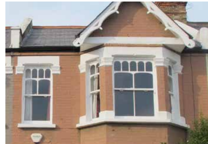
Edwardian hybrid sash window in projecting canted bay, with arched apertures in the upper sash
