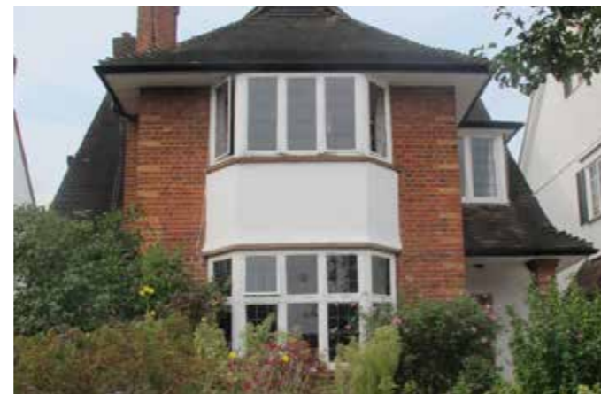
Edwardian Arts and Crafts-style leaded casement windows in the timber-frames of a projecting canted bay, under a low eave
