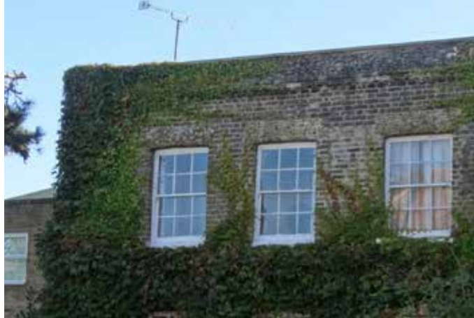
Georgian-style six-over-six sash windows, here featuring 'horns' typical of later sash window styles
