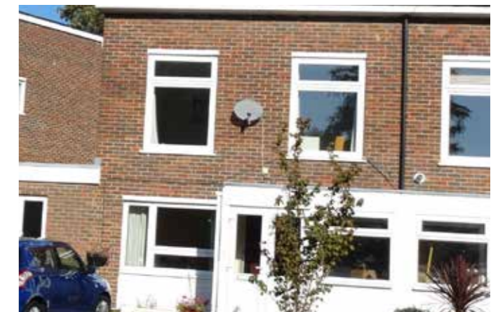
Post-war uPVC windows: with high transom (above) and picture window-form (below)
