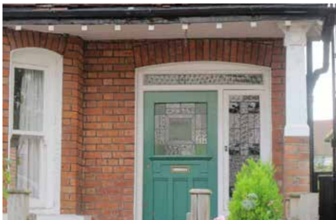
Edwardian narrow sash in a canted bay and, around the door, leaded stained- and textured-glass side light and transom light
