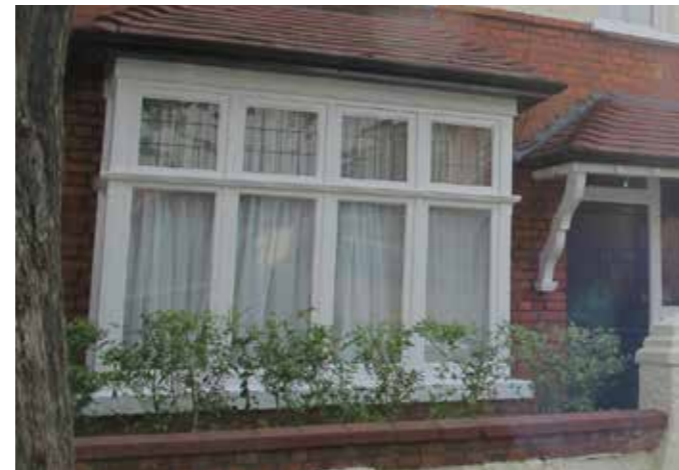
Edwardian projecting square timber bay windows with casement opening and leaded transom lights
