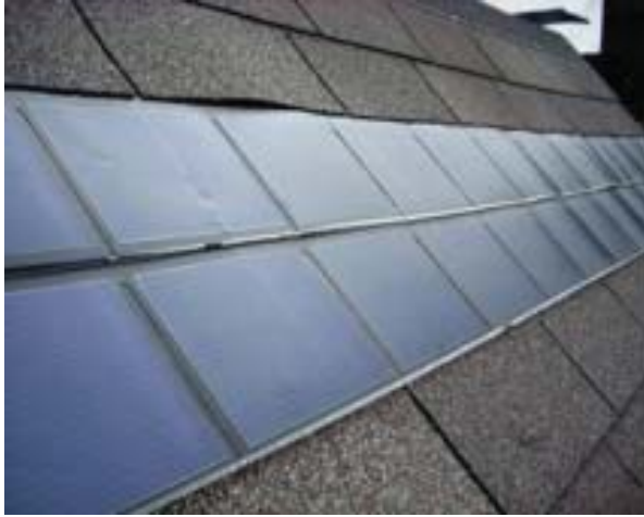
Image 34: Integrated solar panels
