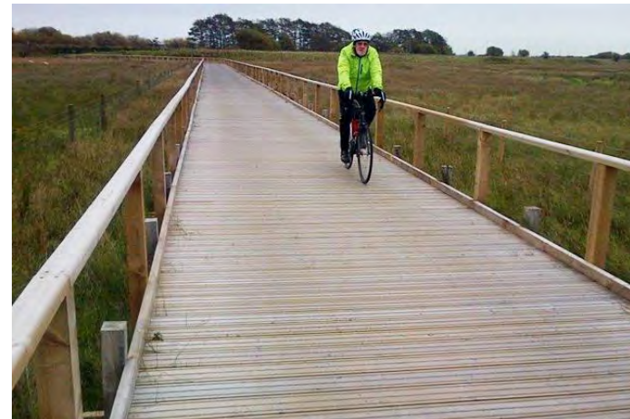
Figure 5-11: Cycle friendly boardwalk – anti-slip decking boards
