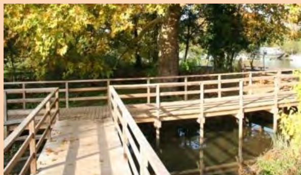
Example of a TLS dry route (upper image shows the site before works were carried out)
