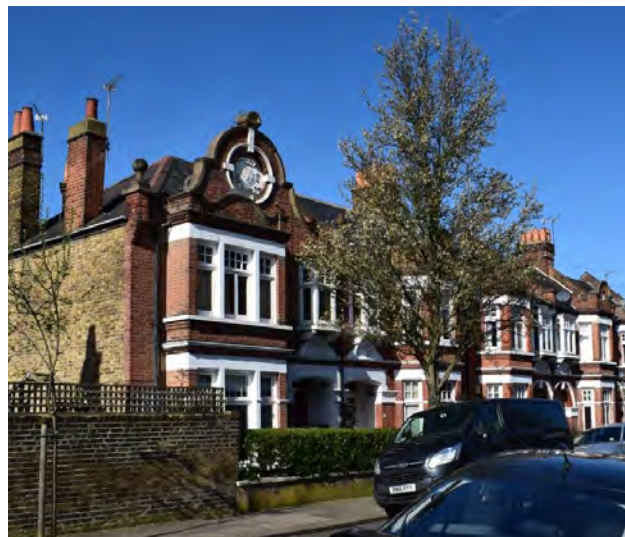
End of terrace in Cowley Road with prominent gable decoration, chimney stacks and hipped roof.
