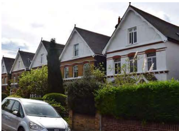
Gabled roofline in Oxford Road with front boundary hedges and brick walls.
