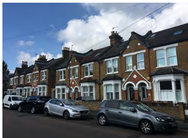
Row houses in Connaught Road with contrasting entrance detail adding interest to the façades.
