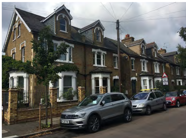
Row houses in Anlaby Road with original dormers and fenestration. The corner house has a double façade.
