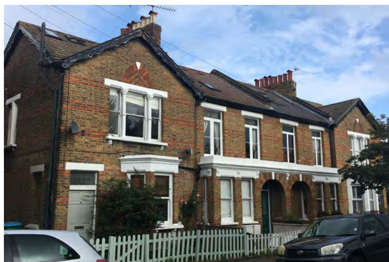
Houses in Royal Road with contrasting brick detailing, integral projecting porches and bays, and low boundaries.
