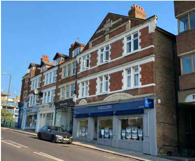
Broad Street buildings leading up to the railway bridge.
