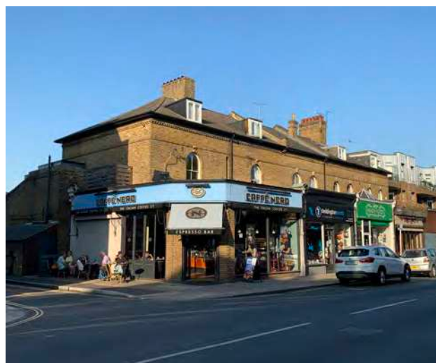
Buildings of Townscape Merit showing historic dwellings behind with single storey shopfront extensions to the front.
