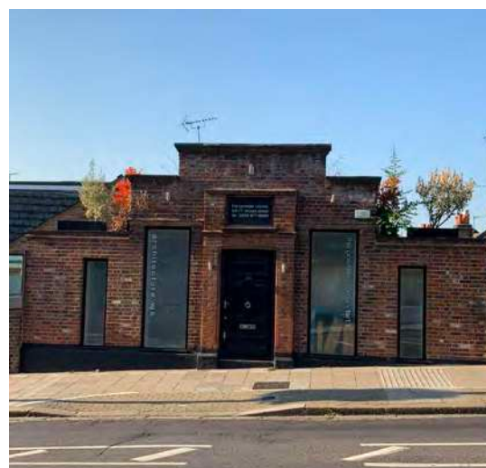
Former public toilet block now converted to offices with additional windows.
