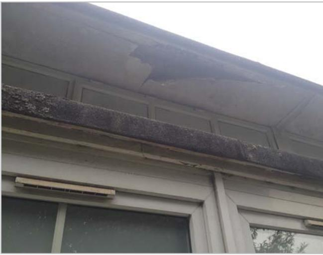
Photo 7 - Hole in soffit
