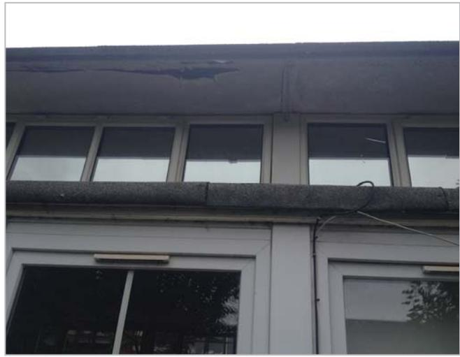
Photo 8 - Hole in soffit
