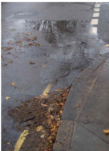
Figure 3-2 Surface water flooding at junction of Amyand Park Road and Strafford Road caused by leaves partially blocking a drain, 25 th December 2007
