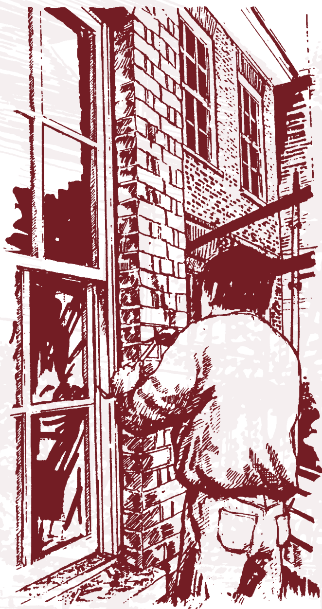
Tuck pointing being carried out to 'The Green' Hampton Court
