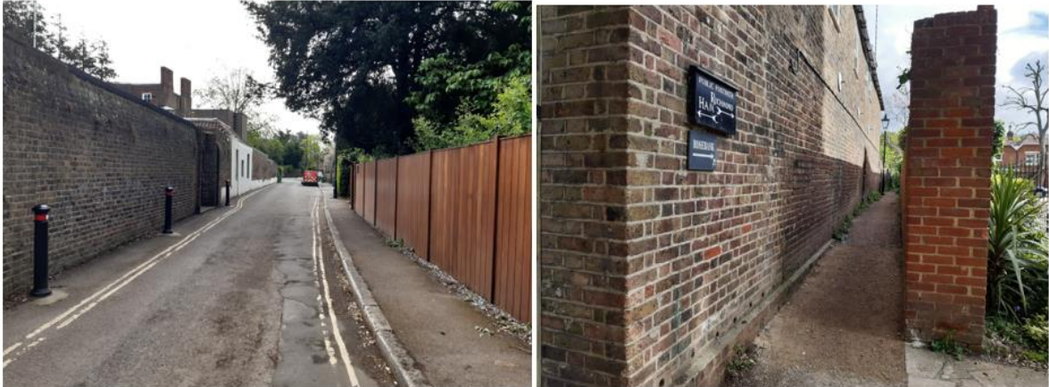
Figure 4: River Lane –mainly used by residents in the area and historic alleyway from River Lane leading to the appeal site.
