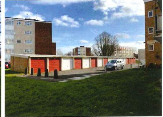
V6. Hornby House Garages
