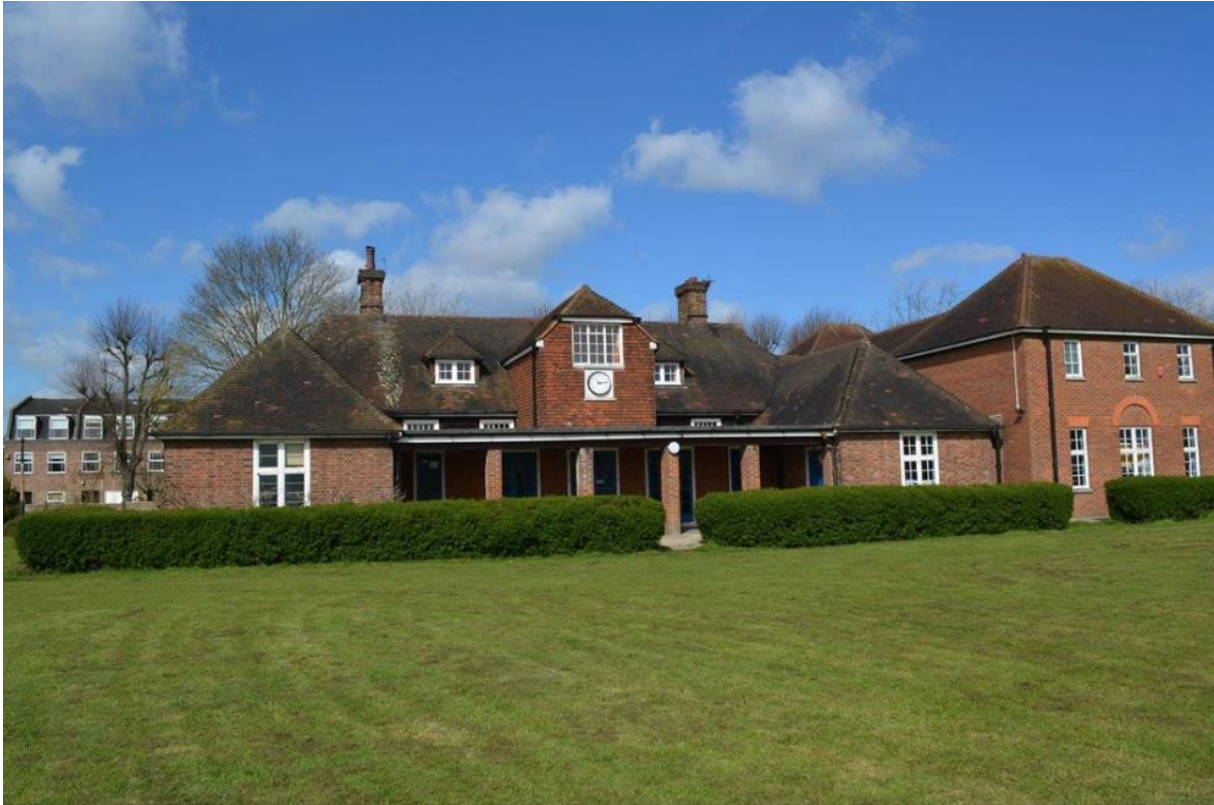
Figure 1 Pavilion. To the left is the original Pavilion opened in 1922. To the right is the second Pavilion added in 1965 (2014 condition)
