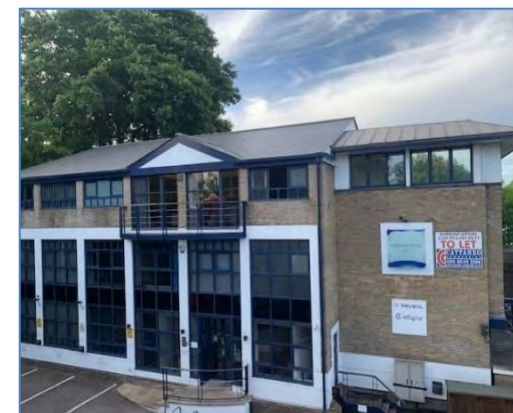
Office Adjacent Kingston Bridge
