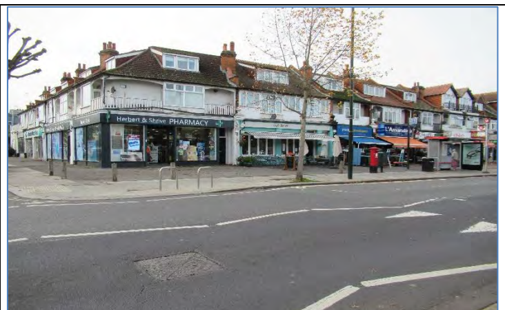
Bushy Park Road section
