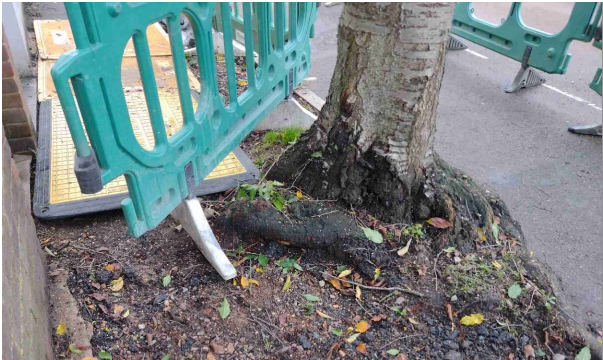
Image shows exposed damage roots at base of trunk obstructing pavement access.
