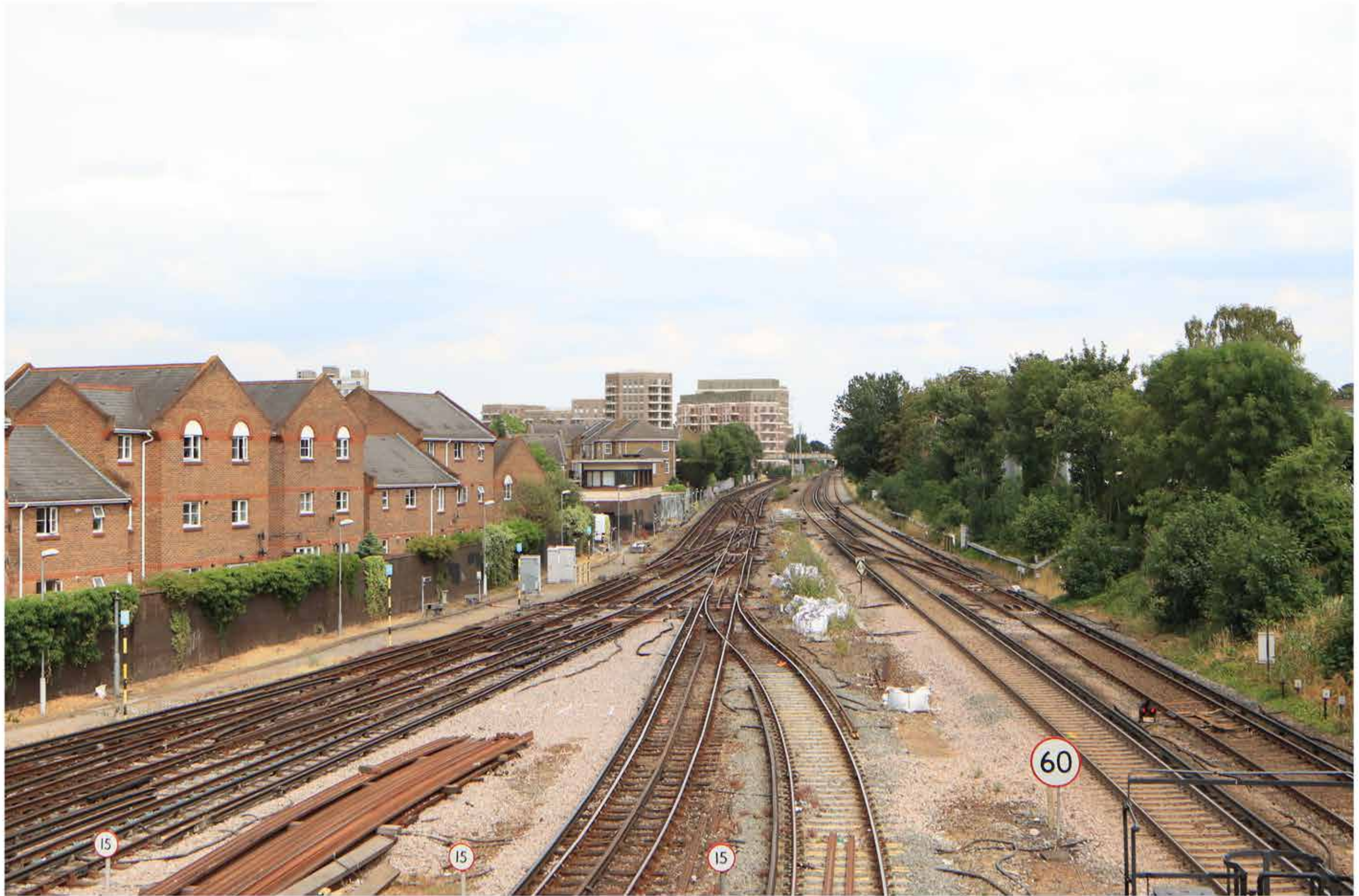
Representative view 5 - Proposed Situation (Amended Proposed Development) A3 with A4 crop marks
