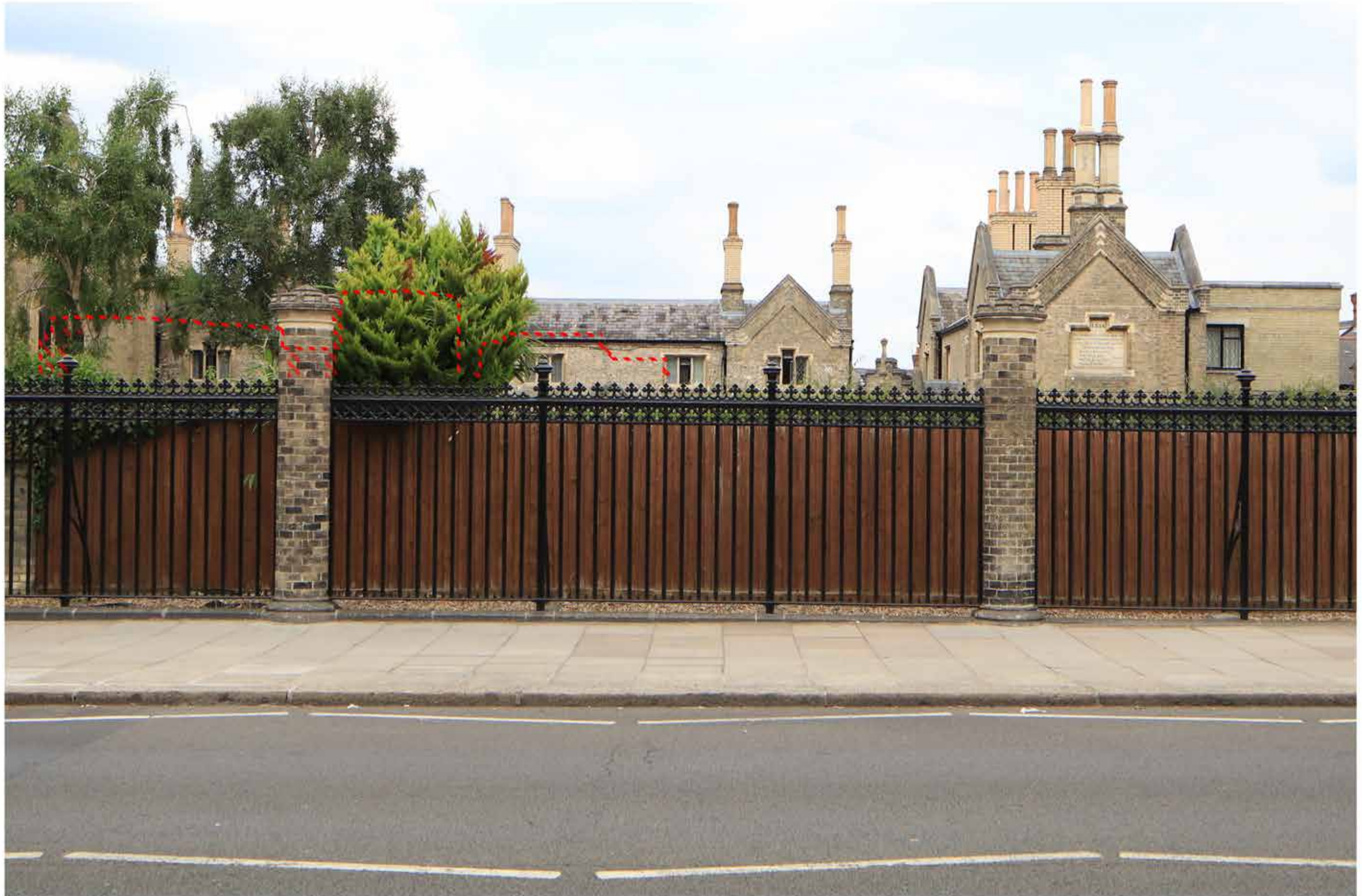
Representative view 3 - Proposed Situation (Amended Proposed Development) A3 with A4 crop marks
