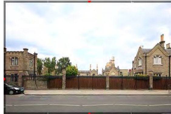
VP 03 - Sheen Road, over Hickey's Almshouses LI - Type 4 LVMF - AVR Level 1
