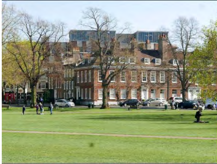
Figure 6 View from Richmond Green Existing 80 George Street with Heritage Assets in foreground, 2020
