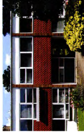
Parkleys Span Housing - Eric Lyons Clay tile hanging
