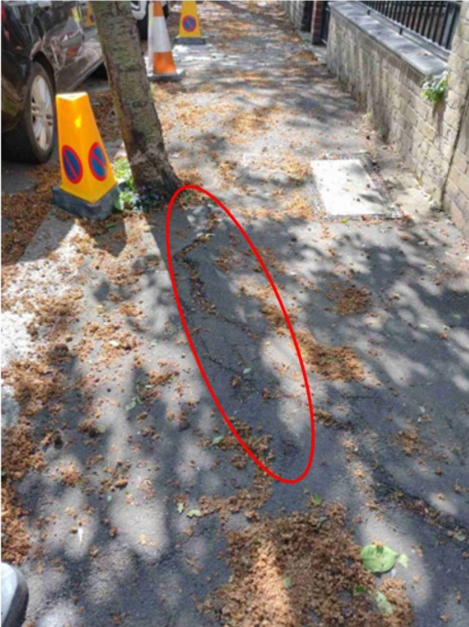
Image shows cracking in pavement surface caused by heave from roots.
