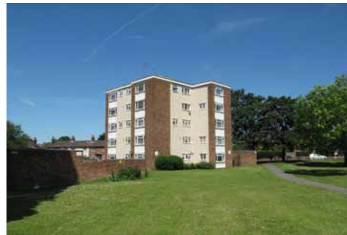
Site photograph 1: Five storey blocks
