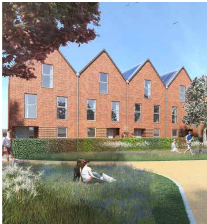
Example of townhouses on the green
