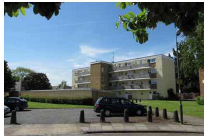
Site photograph 2: Five storey blocks
